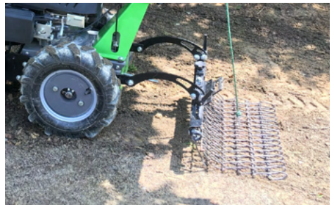
Finishing raking and harrowing
